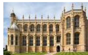
St George's Chapel exterior
